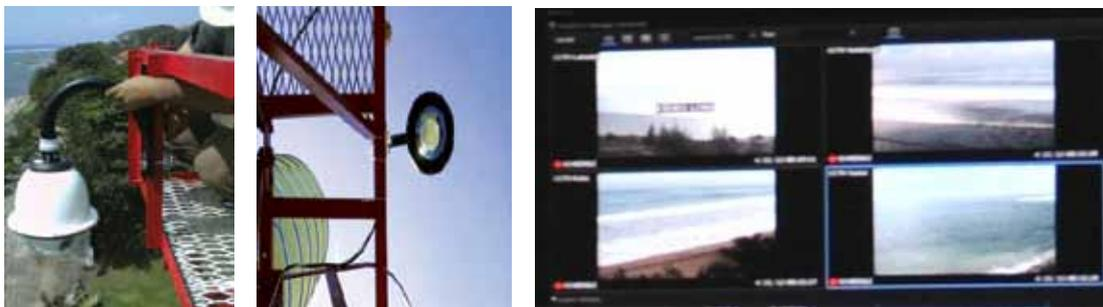
Figure 18: CCTV cameras fitted for tsunami monitoring
